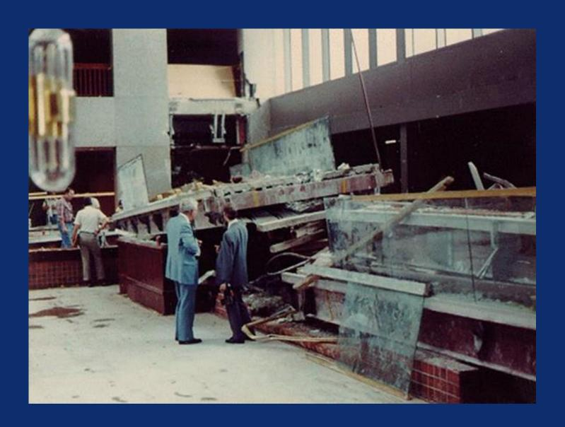
Design change suggested by contractor during construction for ease of fabrication.
